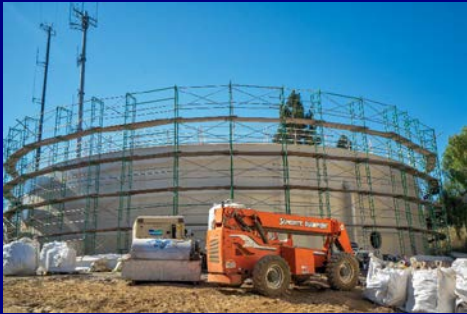
Cadwallader Tank Exterior
