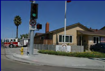
Major Repairs at Fire Stations 18 and 23
