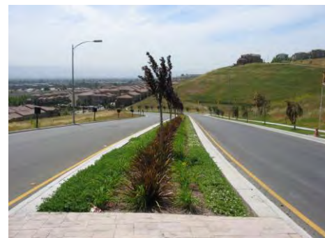
Median Island at Communication Hill
