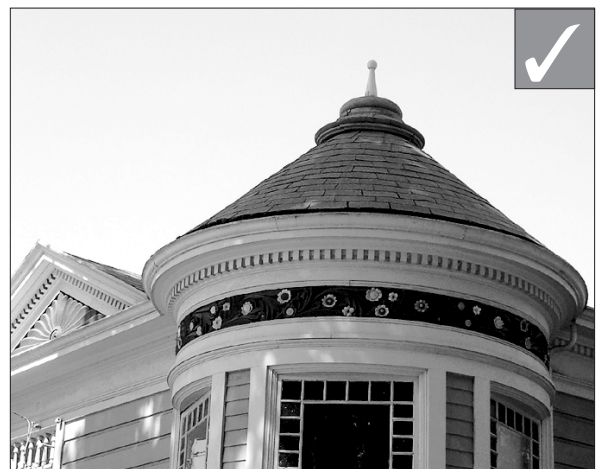
Protect and maintain significant stylistic features, such as these windows, dentils, the flower patterns and the cupola.
