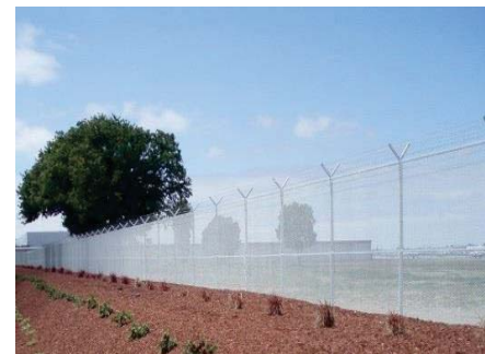
Perimeter Fence Line Upgrades
