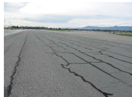
Southeast Ramp Reconstruction
