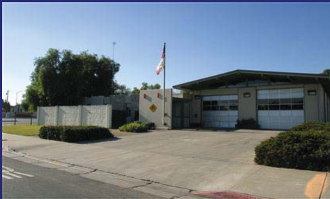
Fire Facilities Remediation
