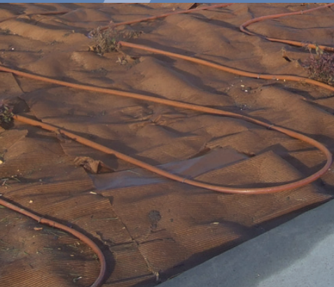
Lay down drip irrigation before adding mulch.
